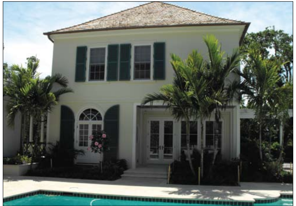
Dobbs After - Finished renovation of demolition shown in previous picture, completed by Croom Construction in 2009.
