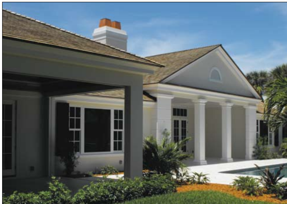
Minton after - Finished renovation of demolition in previous picture, completed by Croom Construction in 2009.
